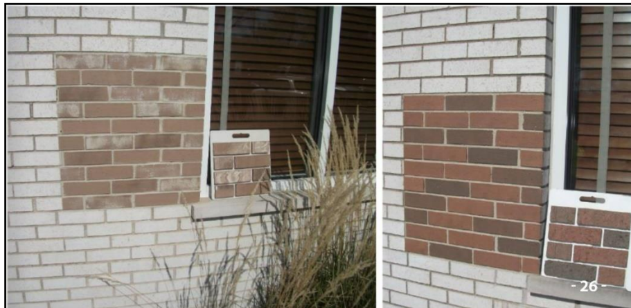
Figure 3 - example of masonry colour transformation using Nawkaw
