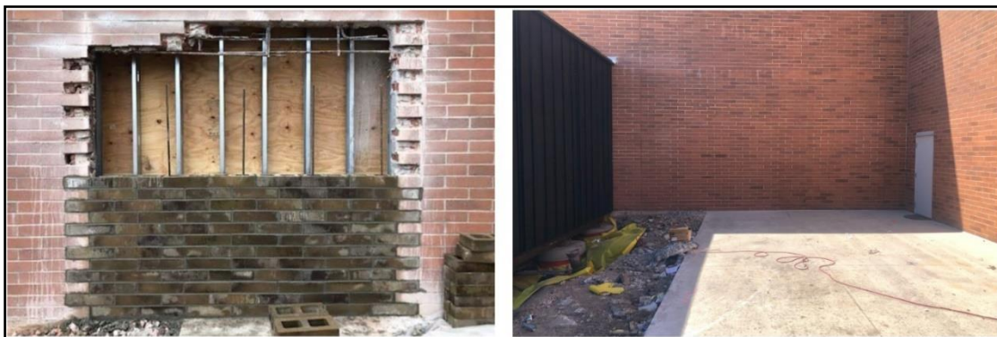
Figure 4 – example of colour matching for masonry infill work
