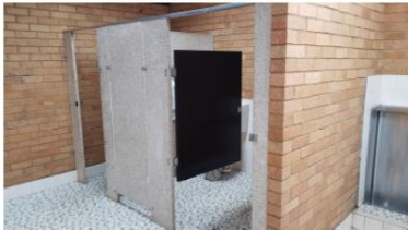
Figure 5.82 South wall – extra pan and non-complying disabled toilet – Adaptive Architects 2020
