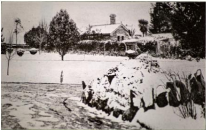
Figure 4.13 The caretaker's cottage in 1908 from the SW looking through what would now be the toilets. Interesting that the rear skillion indicated on the 1891 plan does not appear to be evident, and this image predates later additions. The roof has an iron decorative ridge detail and as it was a residence it was separated from the park with a timber fence. A post and wire fence can be seen in the background - 1908: The Orange District Tourist Guide
