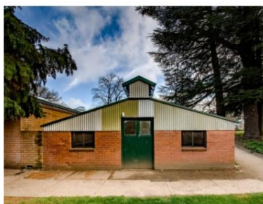
Figure 5.40 The south wall of the c1970 addition to the propagating House. The windows here are different. The corrugated plastic could be replaced with glass – Adaptive Architects 2020
