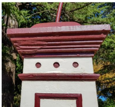
Figure 5.93 Paint falling due to incorrect paint type – retaining water and likely damaging substrate – Adaptive Architects 2021
