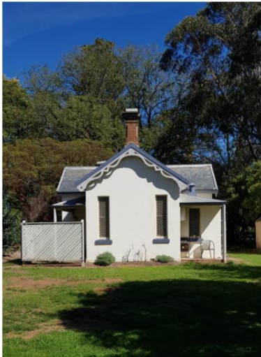
Figure 5.28 The Duntryleague gate house has a remarkably similar plan and the similarities do not end there. It has tall narrow windows, a Classical pitched roof with gable ends, and hipped matching verandah roofs – Adaptive Architects 2021
