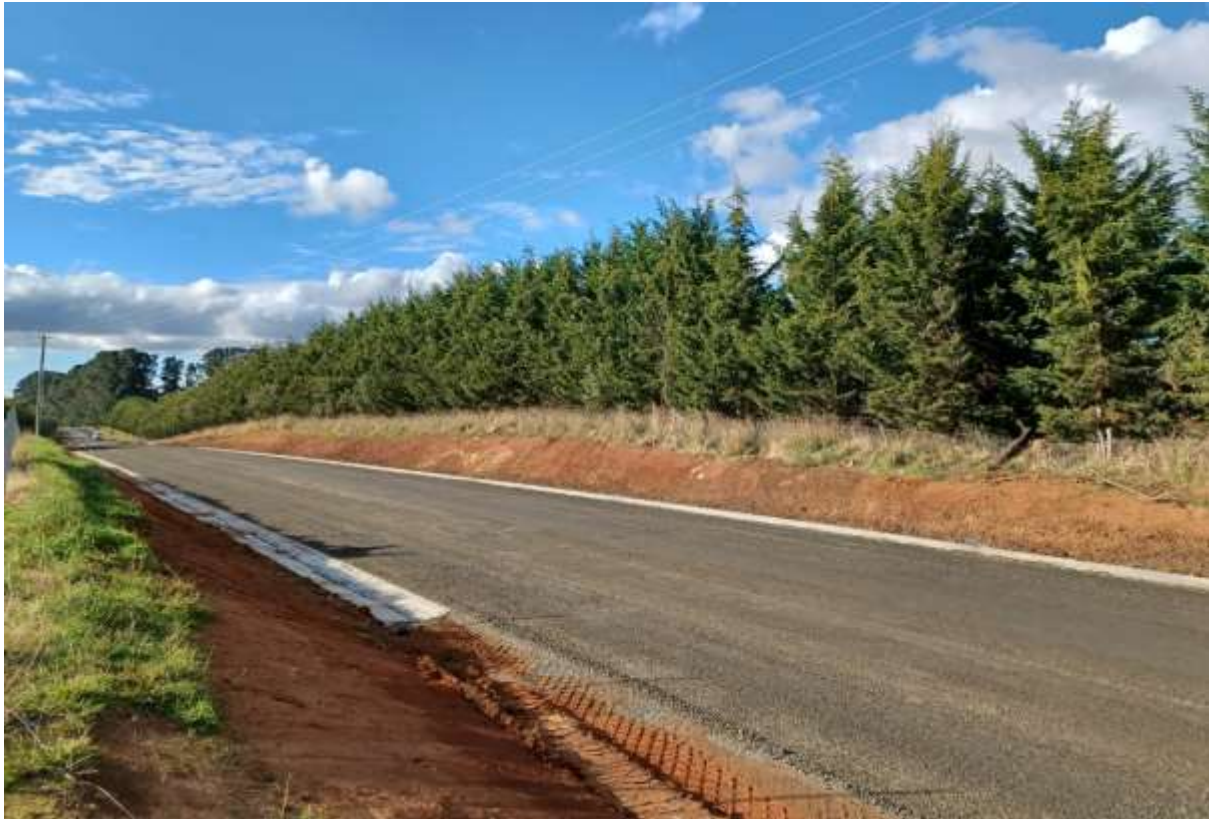
Photo: Crest in Forest Road lowered just north of Hiney Road intersection
