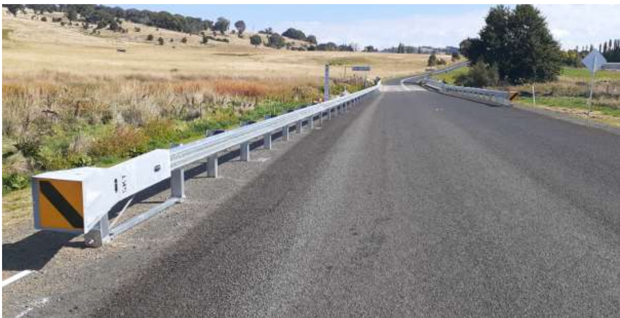
Photo: New guard rail installation on Ophir Road
