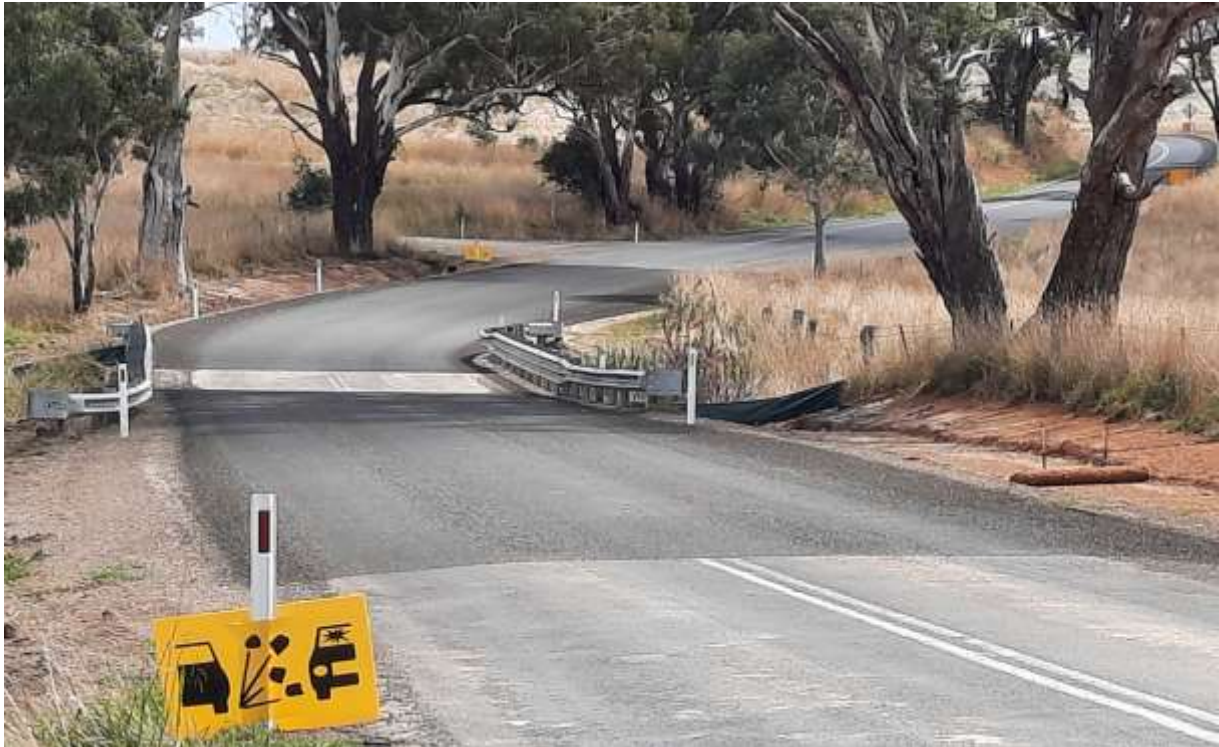
Photo: Icely Road repair to bridge approaches
