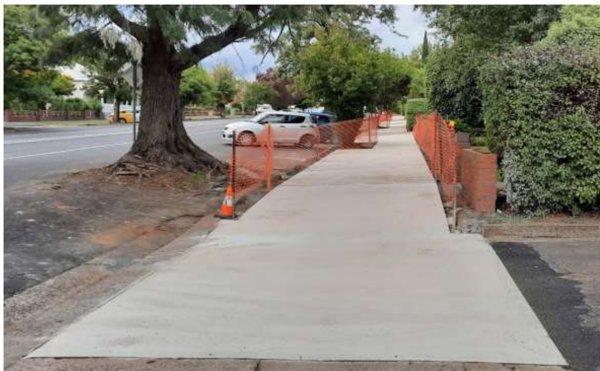
Photo: Footpath reconstruction on Hill Street
