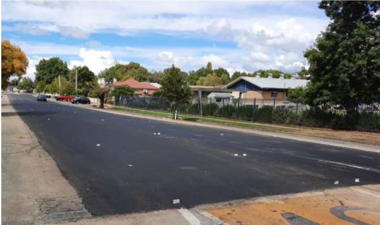
Photo: Freshly laid hot mix asphalt on Moulder Street
