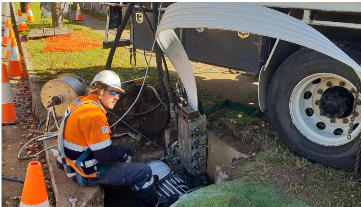
Photo: Pipe re-lining material being fed mechanically into pit for stormwater pipe re-lining
