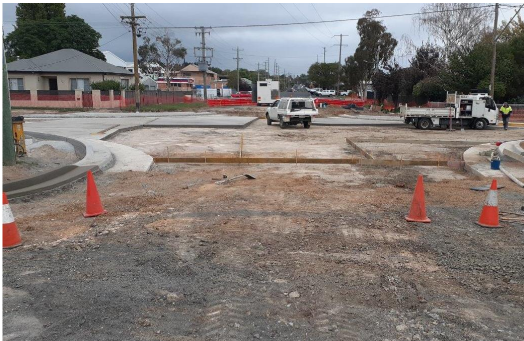
Photo: Progressive forming and pouring of base layers at the March and McLachlan roundabout site
