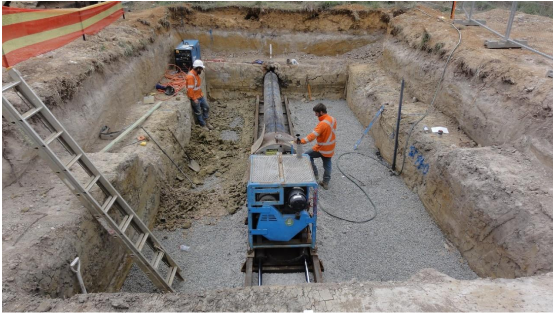
Photo: Railway under-bore
