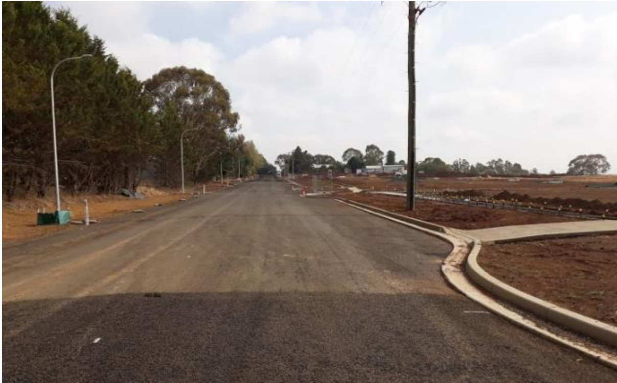
Photo: Shiralee Road sealed ready for asphalt overlay
